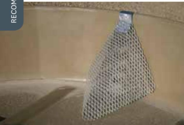
*Birds and other wildlife are drawn to tanks for the valuable water they provide. If an animal falls in, it can swim to an escape ladder, such as this one made of metal screen, and climb to safety.*
